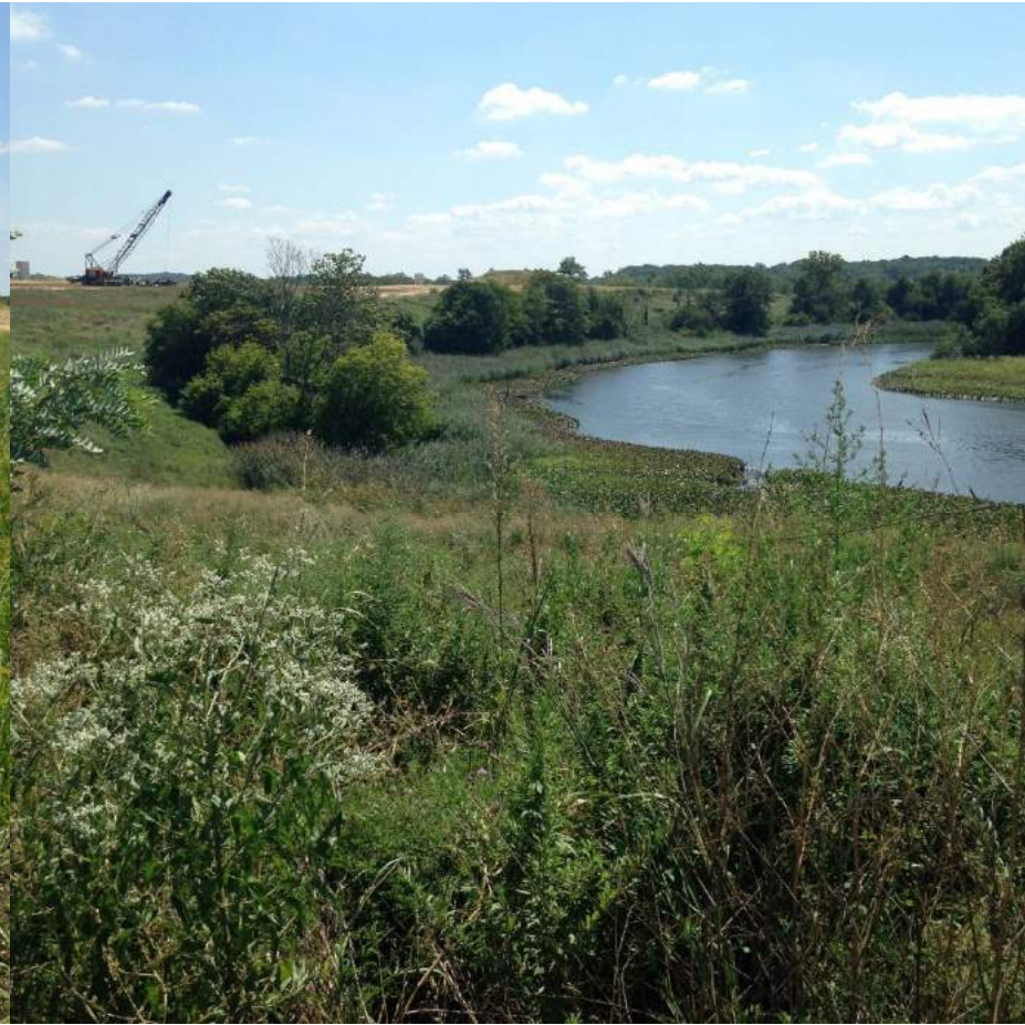
View: Phase I Sideslopes, Big Timber Creek
