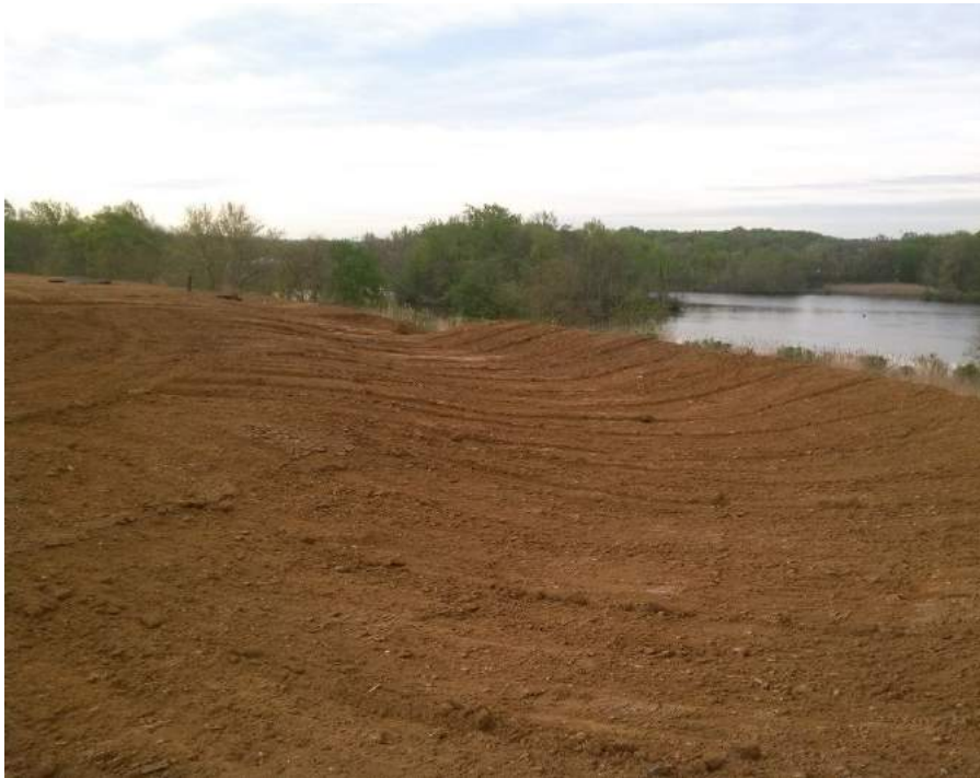
View: Phase I Berms, Lined Swales, South
