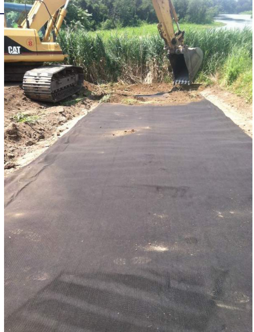
View: Phase I Geodrain Conveyance
