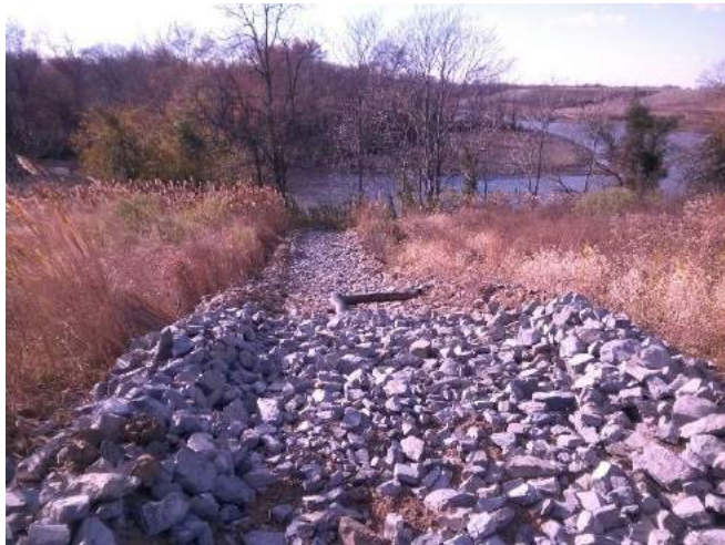
View: Phase I Rip Rap Channels
