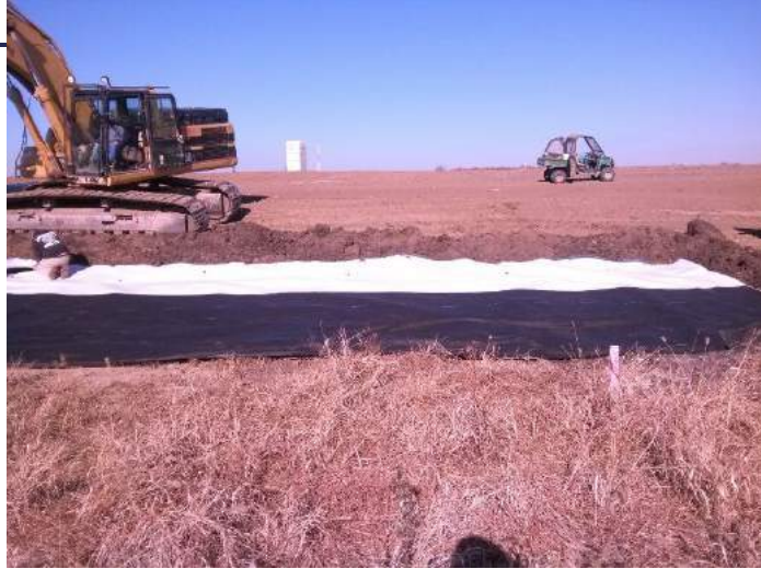
View: Phase I Lined Swales
