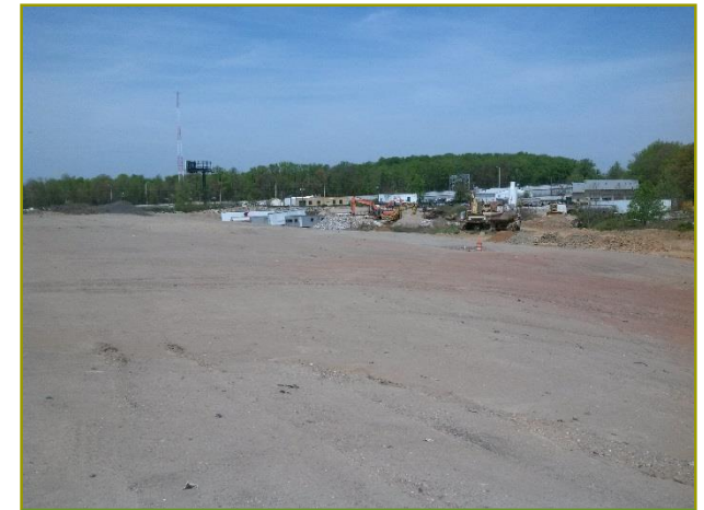
Top of Subgrade
