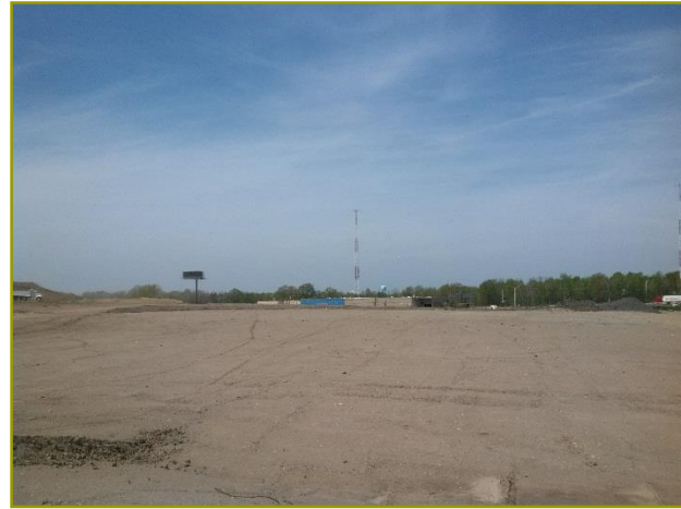
View: Top Facing Creek Road/ NW
