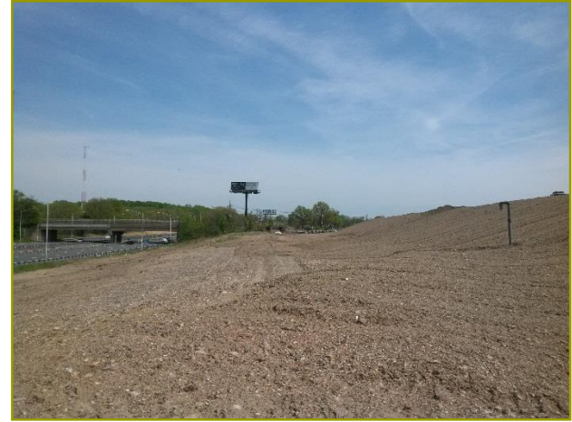
View: Sideslopes Facing Rt 295 S
