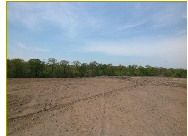
West Corner Sideslopes
