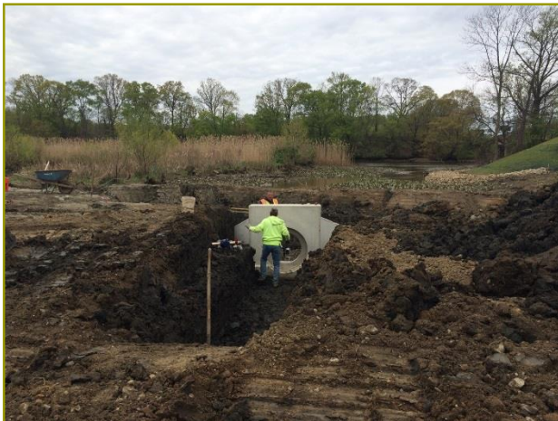
View: Stormwater Pipe Headwall
