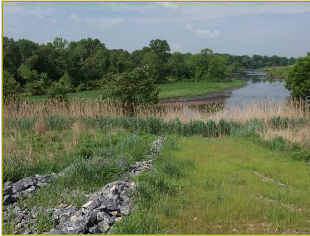
View: Slopes Facing Big Timber Creek
