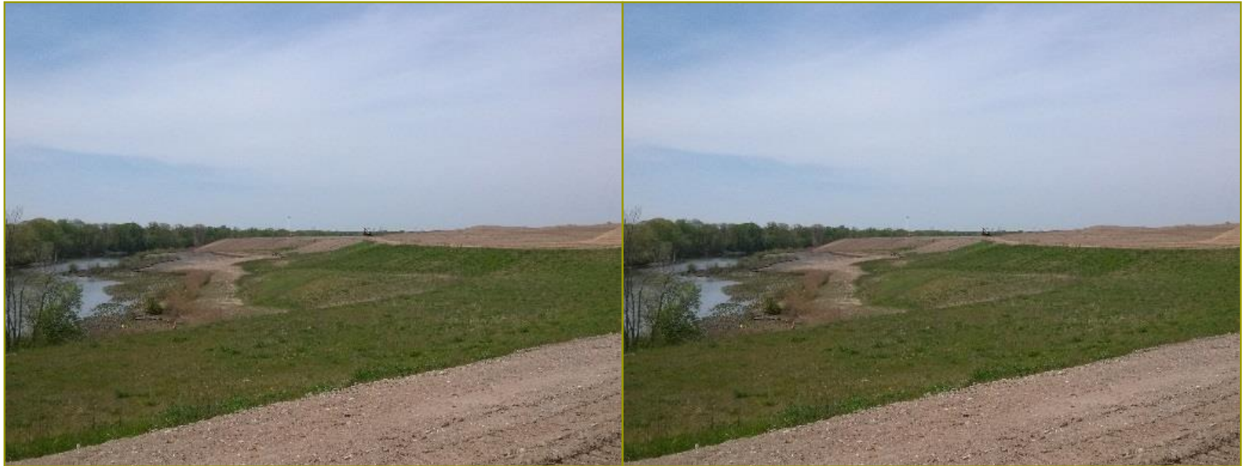
View: Foreground Phase II Slopes, Background Phase III Slopes
