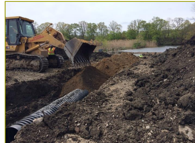
View: Stormwater Pipe Installation
